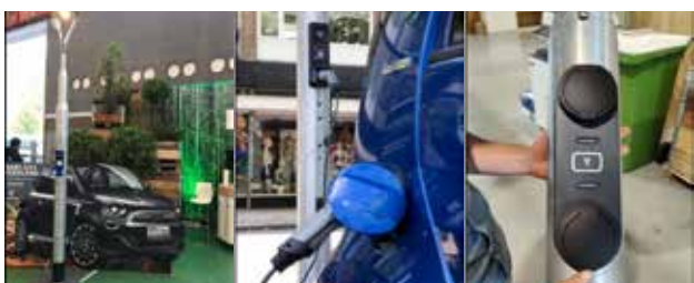
Figure 9: Nedal EV Charging Column:
